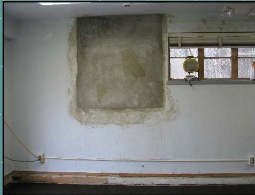
Walls have been repaired and will be painted shortly.
