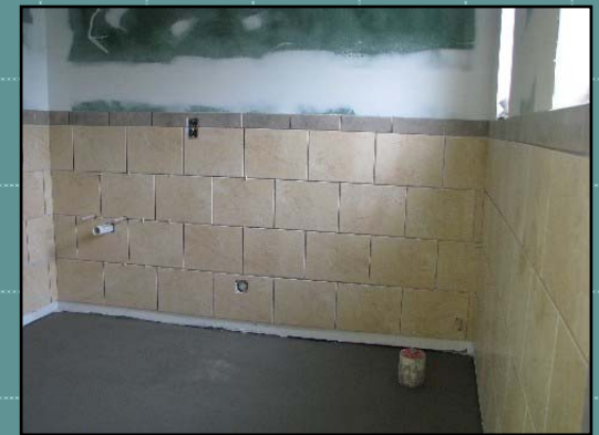
Tiles have been installed in the new handicapped accessible restroom.
