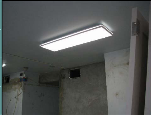
Upgraded lighting system has been installed.
