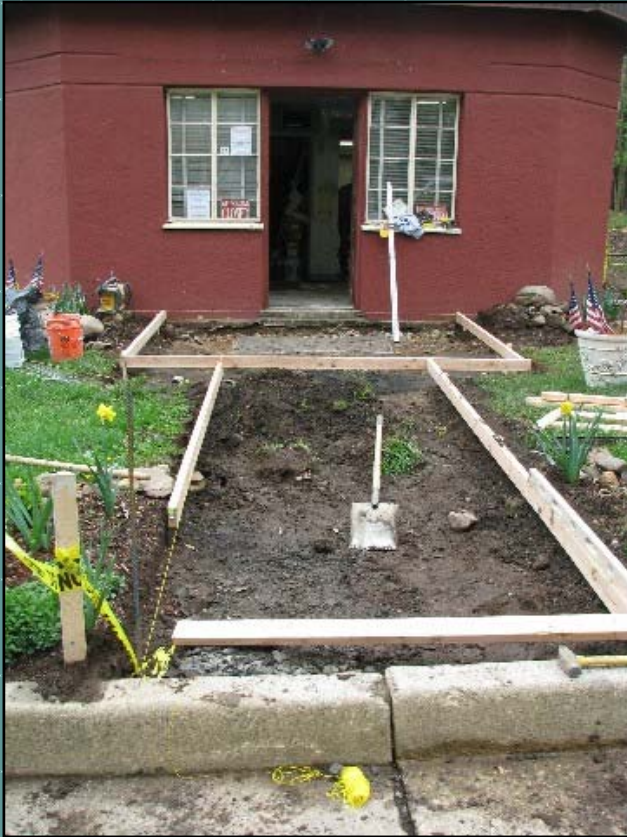
New handicapped accessible walkway has been formed.
